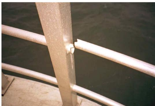
**Figure 8:** The distance between the posts in the fence has been too large creating vibrations caused by the wind. The repair is simple.
